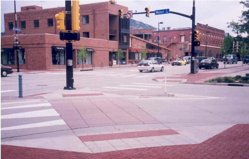
Raised crosswalk condition at an intersection in Boulder, CO that allows wide turning movements while giving priority to the pedestrian.
