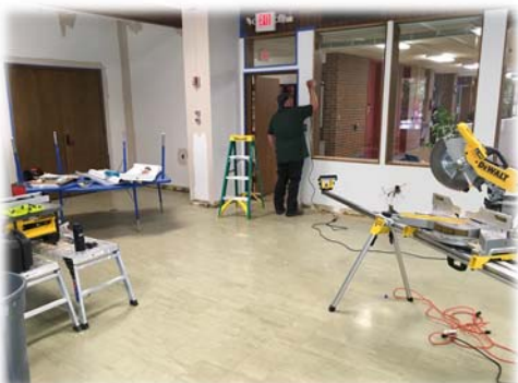
Community Activity Center Renovations
